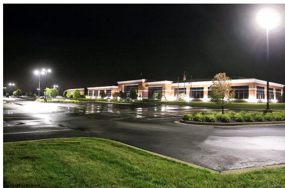
Outdoor car parking lot
