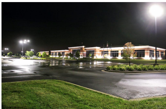
Outdoor car parking lot
